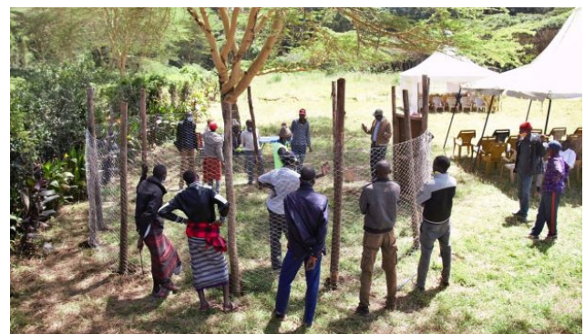
Demonstration boma built by trainees.
